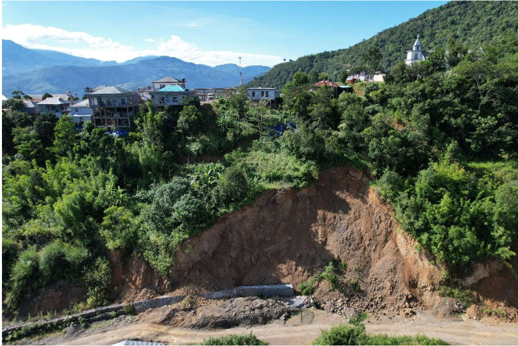
Fig. 4. Landslides near Melbuk village after infrastructure works & heavy rainfalls
