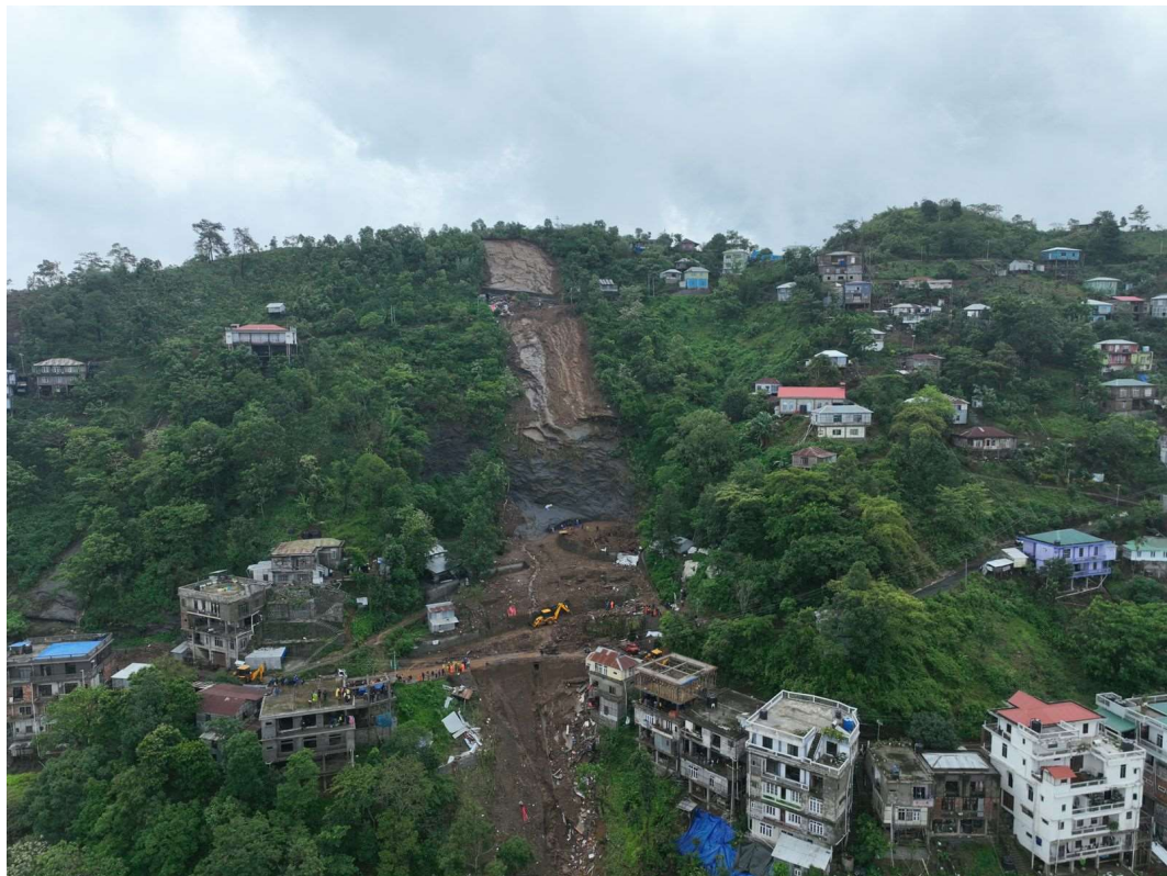
Fig. 5. 16 persons killed at Melthum landslide after Cyclone Remal; damage and loss assessment done by the Centre for Disaster Management, Mizoram University
